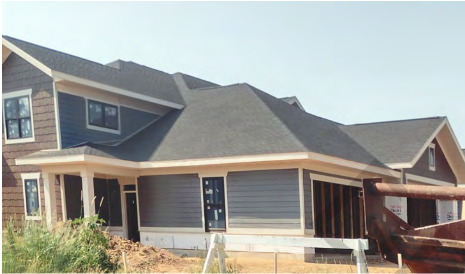
Construction of new single family homes
