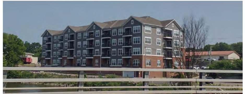
Newer high-density apartment complex overlooking the Baraboo River
