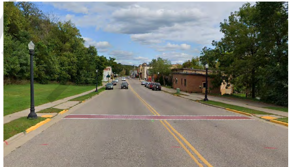
Marked crosswalks increase visibility for pedestrians.
